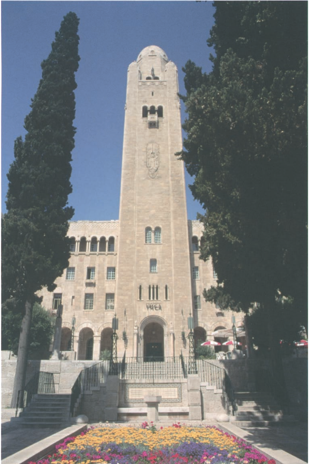
The YMCA building in West Jerusalem, across the street from the King David Hotel. © Hanan Isachar/CORBIS
